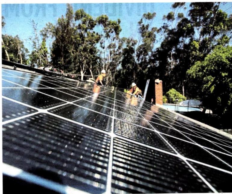
Solar installers placing solar panels on the roof of a house. It is now possible to provide reliable and affordable electricity via rooftop solar systems without a central power plant or transmission and distribution lines. REUTERS PIC
